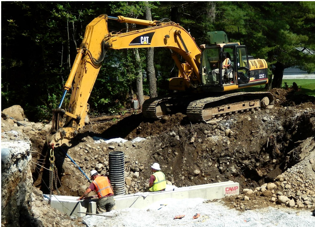
Spring Lake Road Box Culvert Replacement
