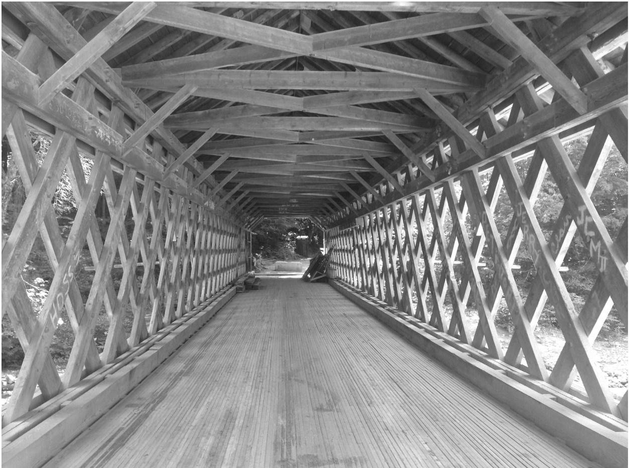
Interior of Brown Bridge during lattice work repair.
