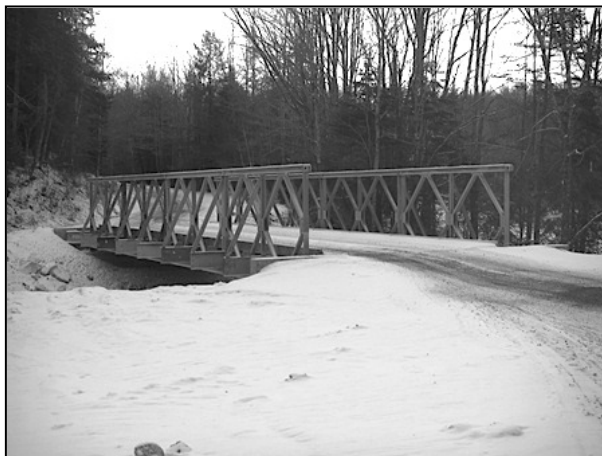
The temporary Frank Lord Bridge—a quick welcome repair after the flood.
