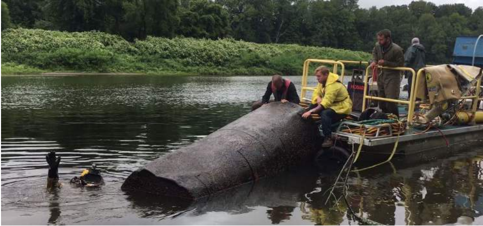
Fuel tank being removed from the Connecticut River.
