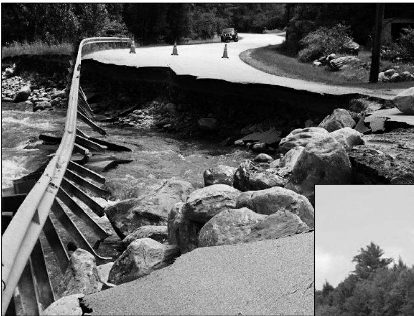
Flood damage to Cold River Road (above) and some of the rocks needed to repair it (right).
