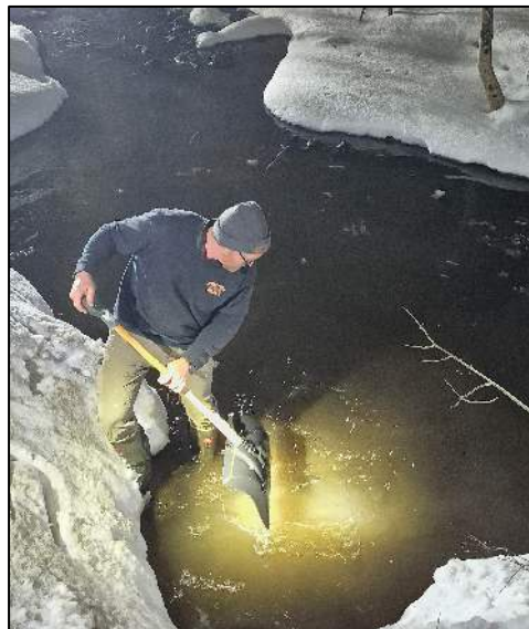
Chief Phil Severy clearing debris from a dry hydrant intake.
