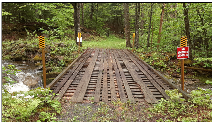
The bridge we want to replace and move to straighten the trail.
