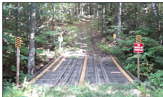
A bridge on 407 that was repaired last year and was inspected this year to see if it was still good; It is good for another year!
