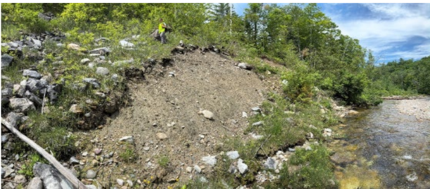
The “lower unit” of the eroded embankment near Cold River Road, with a geologist for scale above the exposure. Larger boulders on the surface to the left in the image were placed as riprap sometime after 2011. Photo Credit: VT Geological Survey.
